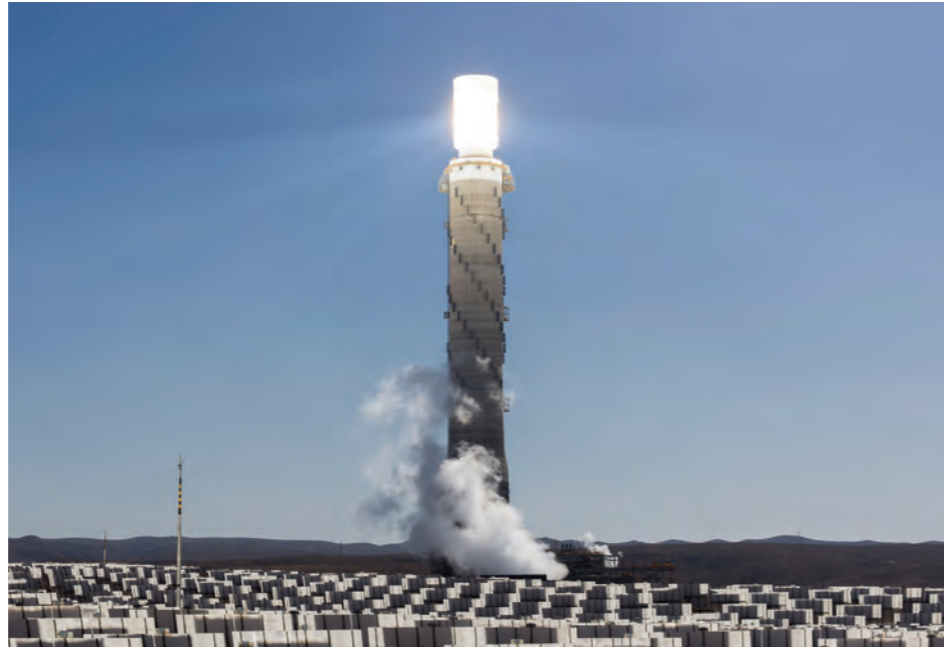
The MST team is utilising the vast expertise of the SZMF R&D institute for projects ranging from solar power to fertilizers.
